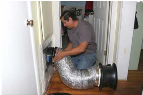
Duct Blaster Test
